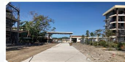
Land and Road Network Improvement of San Isidro Extension Campus
