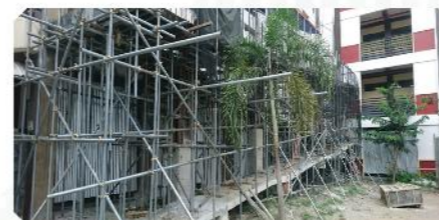
Construction of CCS PWD Ramp
