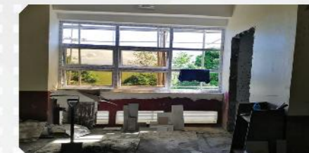
Rehabilitation of the College of Education Building
