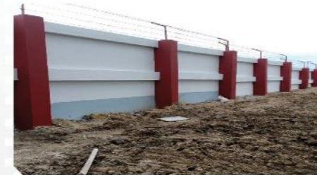
Rehabilitation of Fence at Lucinda Campus
