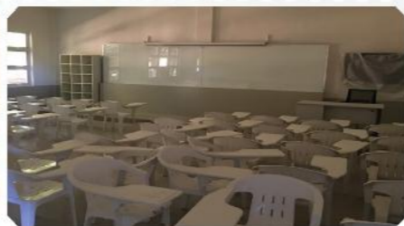
Refurbishment of Classrooms and Laboratory Rooms (Phase IV) College of Engineering and Technology Building
