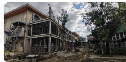
Rehabilitation/Renovation of Academic Building – College of Architecture and Fine Arts Building
