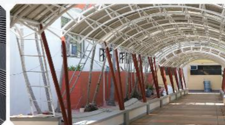
Replacement of Covered Pathway located at Main Campus
