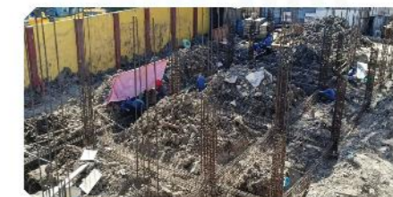
Construction of Three-Storey Administration Office and Motorpool Building (Phase I)
