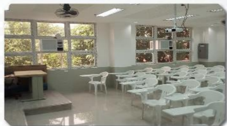
Refurbishment of Classrooms and Laboratory Rooms (Phase III) College of Teacher Education
