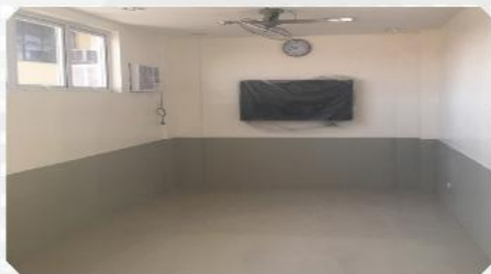
Refurbishment of Classrooms and Laboratory Rooms (Phase IV) College of Public Administration and Governance Building
