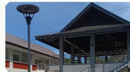
Rehabilitation of NSTP Building/Improvement of Academic Building 2- Storey NSTP Building Lucinda Extension Campus
