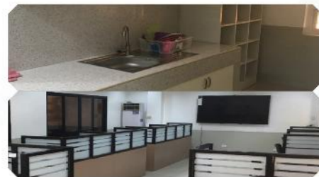
Refurbishment of Classrooms and Laboratory Rooms (Phase IV) College of Criminal Justice Education Building
